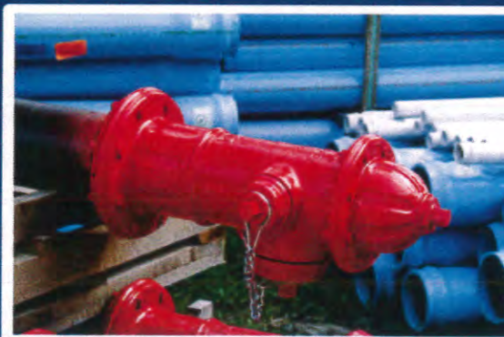
Recently installed water pipe & hydrant in Letcher County, Kentucky.
